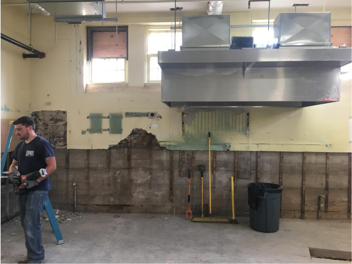
Exhaust hood installed, and plumbing work is moving along. You can see the big trenches to accommodate the plumbing...
